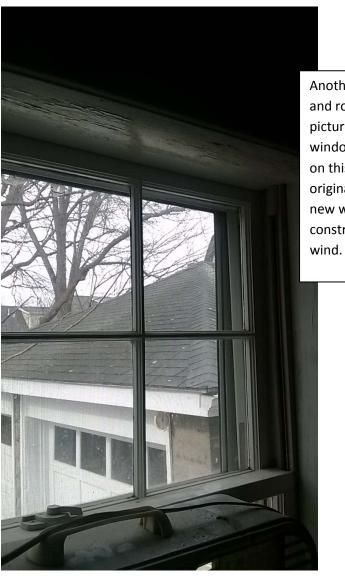
Another west facing window with indication of water damage and rot from water leaking through exterior fascia board. The picture also shows that these are old replacement sash windows and are not original to house. There are no headers on this window...it was just cut into wall and its location is not original to house. We are asking to replace these sashes with new wooden ones that offer double pane glass and better construction and better protection to house from rain and
